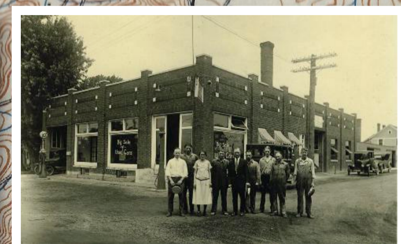
William Emerson Ayer (1893-1936) opened one of the earliest car dealerships in Anderson in 1916. This photo (ca. 1923) includes company employees and the building at the corner of today's Beechmont Avenue and Wolfangel Road.
